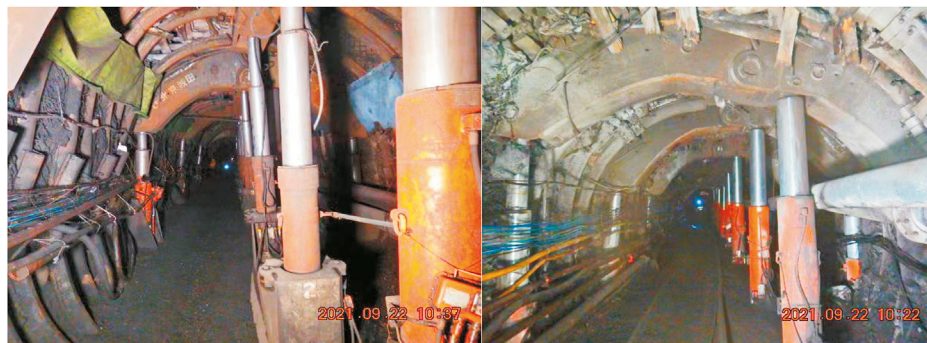
Fig. 20. Application of anti-bursting support in the roadway.
